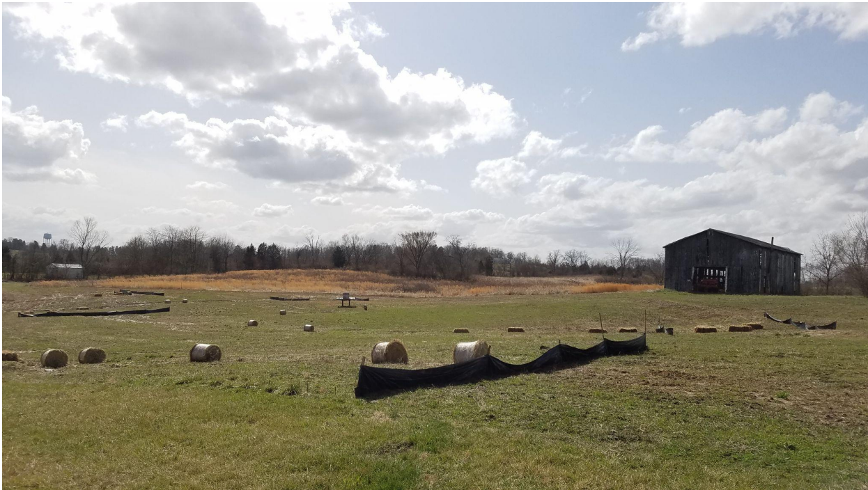
Photo 14 - Installing erosion control measures post-seeding.
